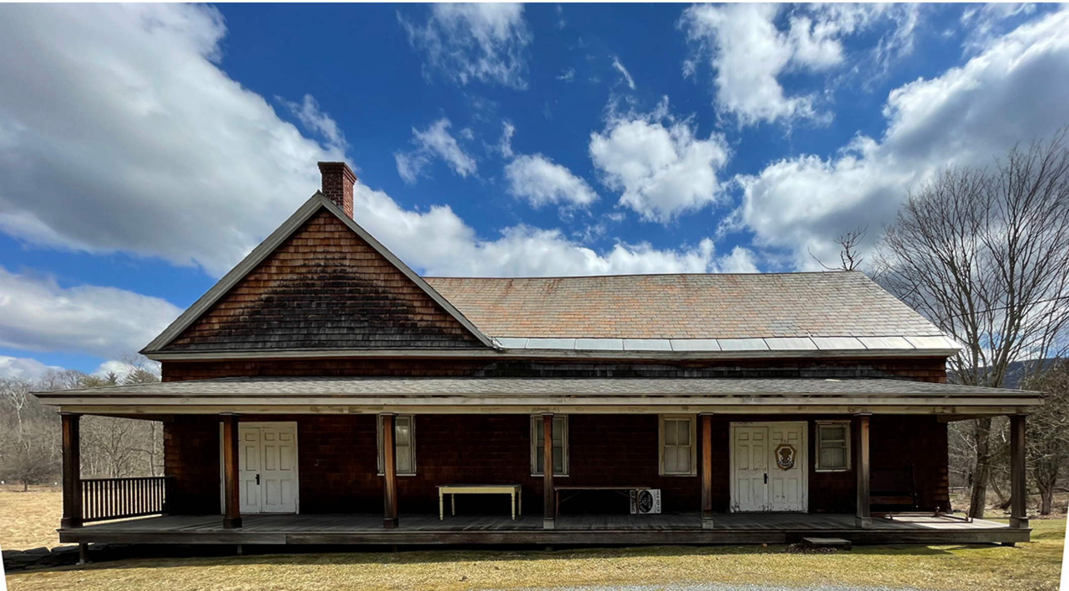
HISTORIC WILLIAMSTOWN GRANGE HALL – RENOVATED AS 5 GROUP 2B FULLY ACCESSIBLE DWELLING UNITS OF WHICH 3 ARE AFFORDABLE.
