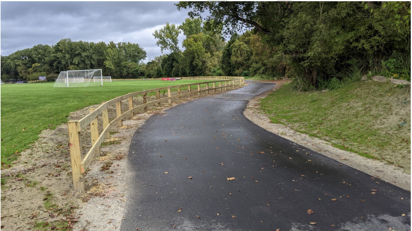
Figure 24: Mohican Trail at Williams Athletic Facilities
