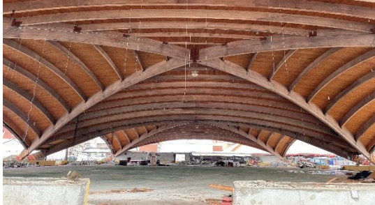
Towne Field House roof structure
