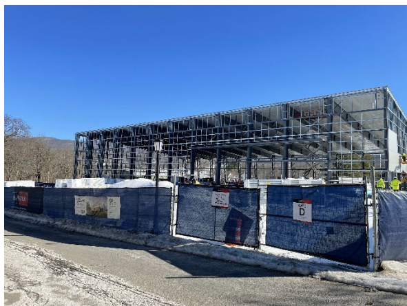
Figure 1: Progress Photo of New Fire Department Building
